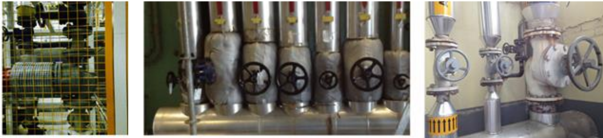
Valvs production (Herdez) – eksempel of insulated valves from denmark – Valvs boiler (Herdez)
